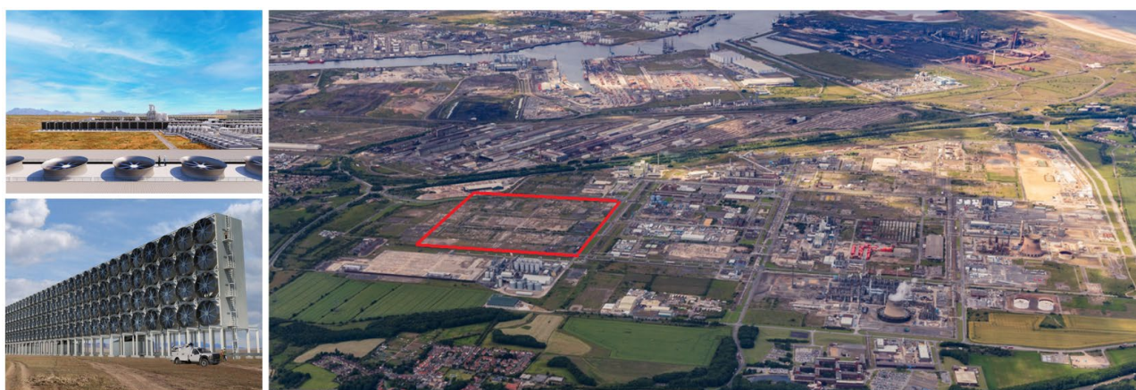
Figure 4.4: Example of size and land requirements for 1MtCO 2 /yr DACCS facility. Top left & bottom left: renders of Carbon Engineering DACCS facility. Renders produced by Carbon Engineering (Carbon Engineering, 2021; Leah Burrows, 2018). Right: Example ~100 acre plot marked out in red at the Wilton International site in the Teesside cluster). Image from Wilton International (Wilton International, 2023).
